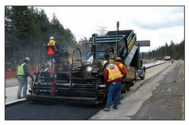
Like a rotating laser, Lazer Zone supports multiple users. Using a PZS-1 sensor and Topcon's FC-200 field controller on a grade rod, basic surveying tasks and grade checking are a snap. In situations where multiple PZL-1 transmitters are being used, each can be set to one of four signal channels. The system will transition seamlessly from transmitter to transmitter without disruption.
